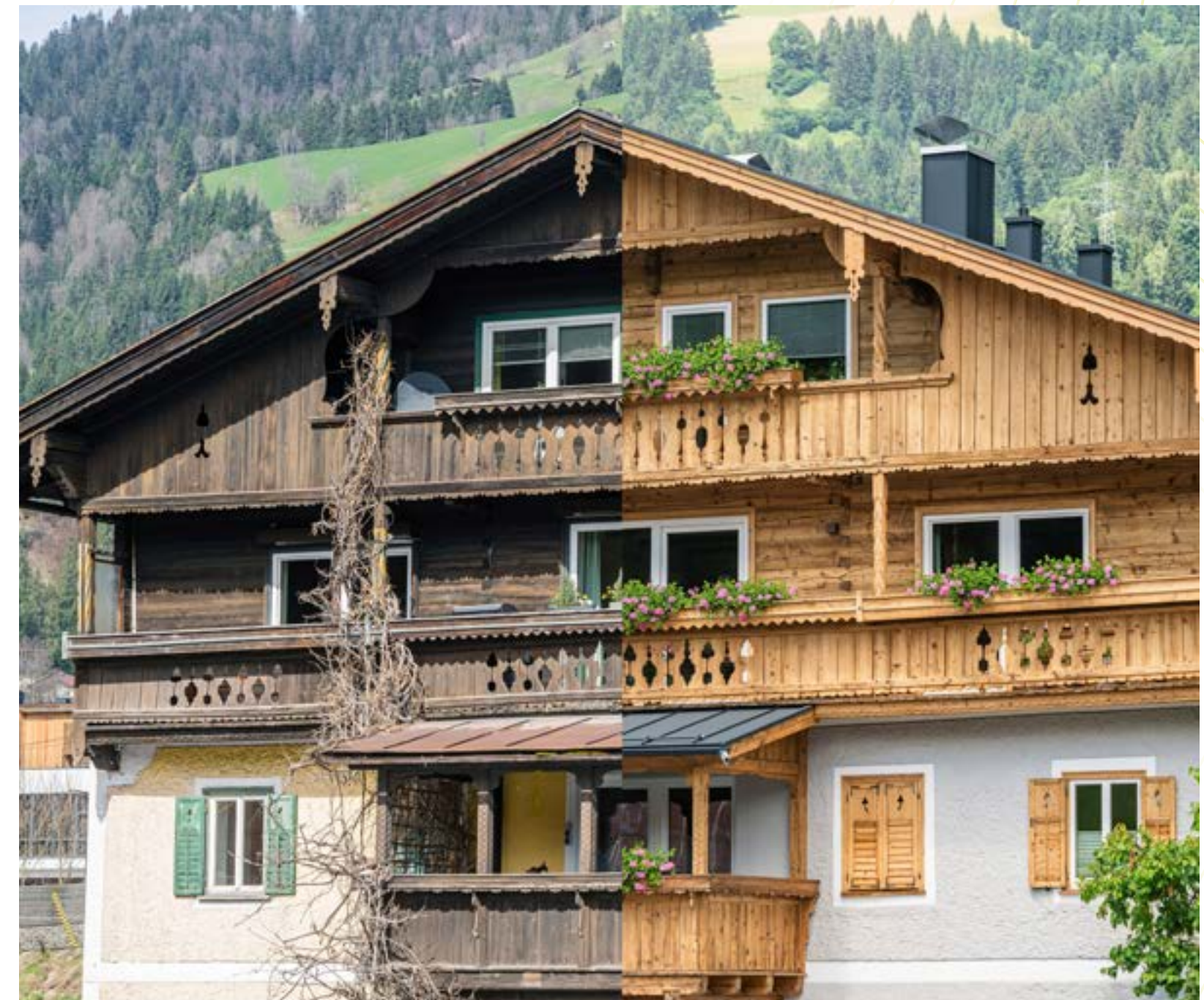
Thanks to the SWARCOBLAST glass blasting granulate, wooden houses look as good as new. Left: Before the surface treatment; Right: After the surface treatment Photo credit: Strahltechnik Lechner GmbH
